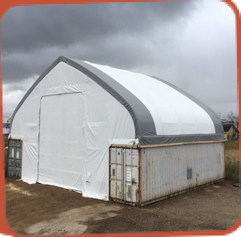
Container Storage Shelter
